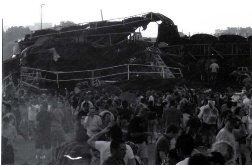
Collapsed stage at Ottawa Bluesfest. Photo: Sandra Luty
